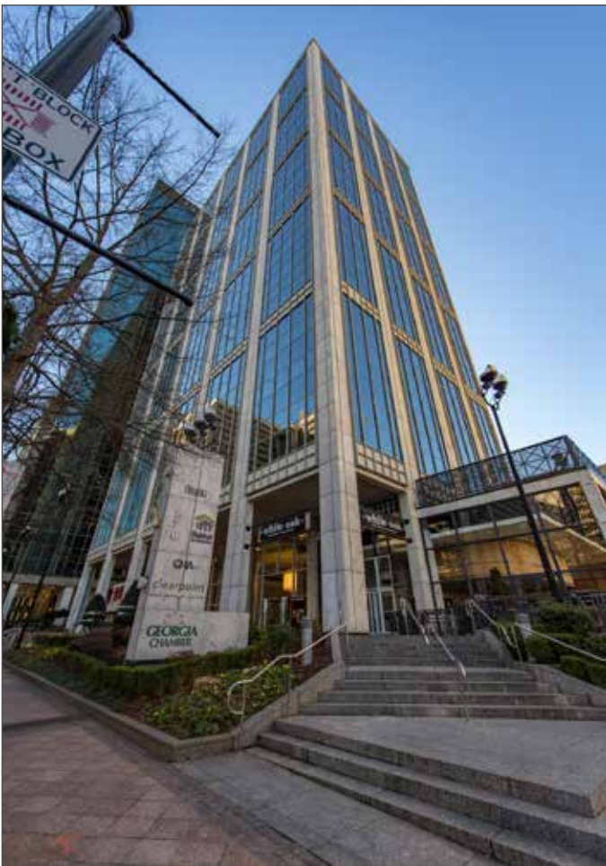
Southern Telecom's 270 Peachtree facility is located in downtown Atlanta
